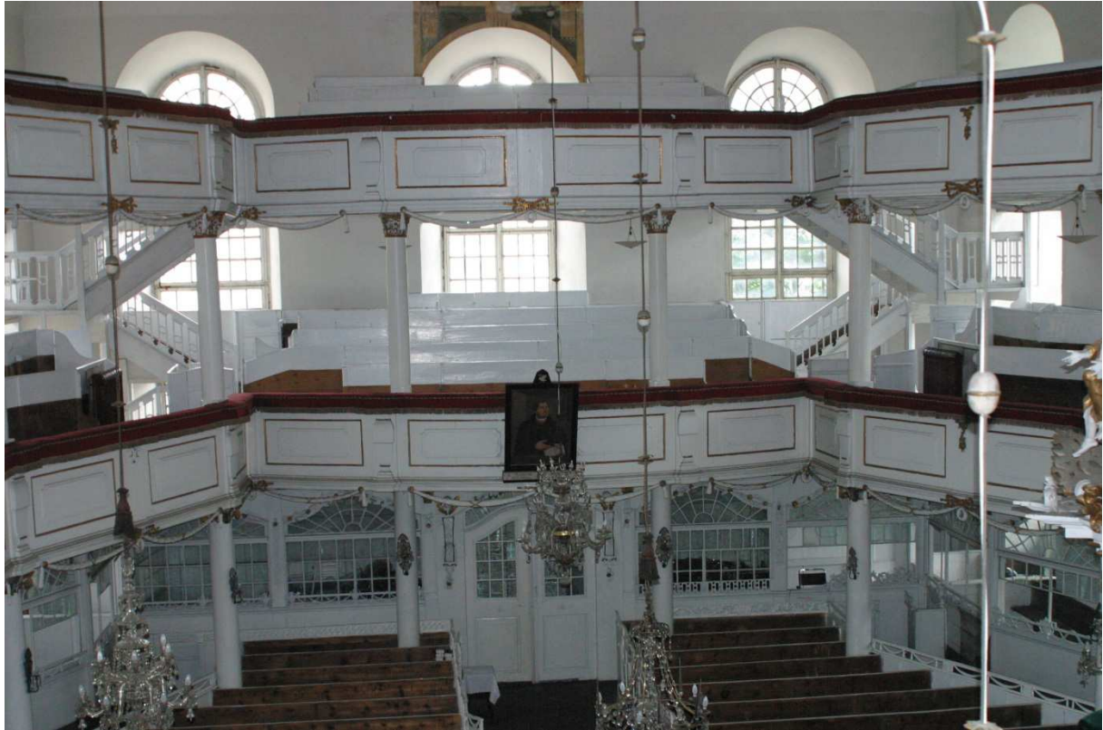
Innenraumansicht gen Westen, September 2011
